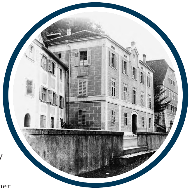
The first assembly venue for Parliament in the House of the Estates (Ständehaus) 1868 – 1905.
